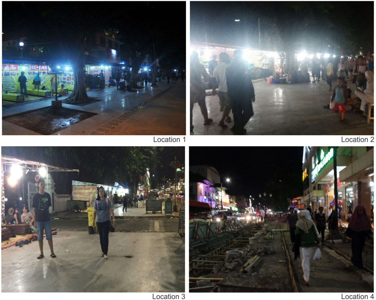
Fig. 2 - Existing condition at nighttime
