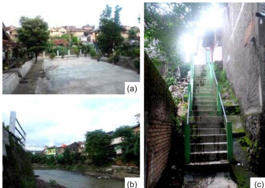
Fig. 1 - Existing condition: (a) Playground area; (b) The cliff and river; and (c) Access to the playground area
